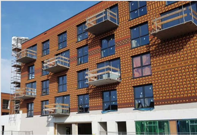
Balconies under construction
